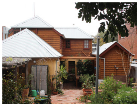
NEWMAN HERITAGE HOUSE REGENERATION FREMANTLE PETER AND JAN NEWMAN WITH GERARD MCCANN
