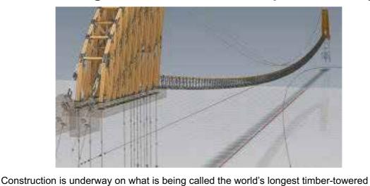
will be completed in June 2022. The 1,203-ft long and 118-ft high pedestrian bridge will span the chasm between the peak of McLouth, near the top terminal of the resort's express chairlift, and end at the summit of Disciples Ridge Credit: Woodworking Network Read more and watch the video
