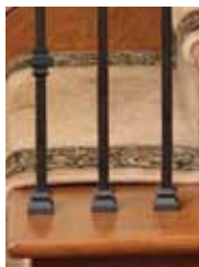
Open Tread Bottom Connection
