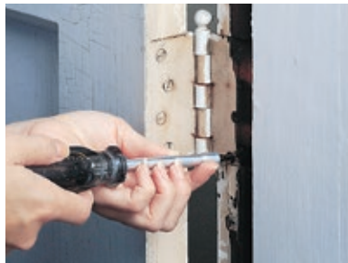
2 Remove the old door, strike plates, hinges and threshold
