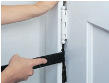
1 Carefully remove and save interior trim
