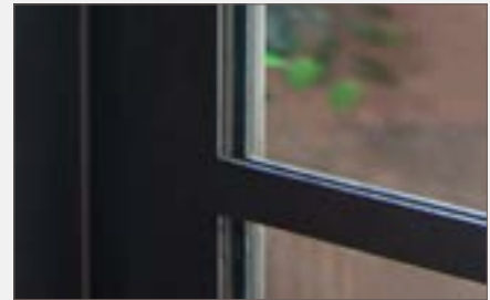
Aluminum glass frame provides a flat minimalist appearance on both sides of the door.
