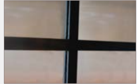
Profiled aluminum muntin bar has only a 1-1/8" width and includes an internal "shadow bar".
