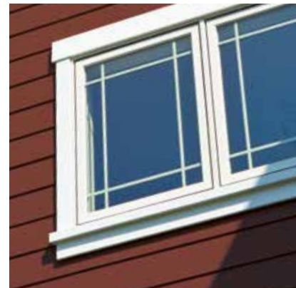
Window surrounds complete the curb-appealing picture.
