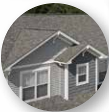
Roofing and Ventilation
