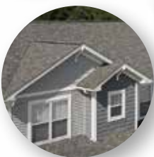
Roofing and Ventilation
