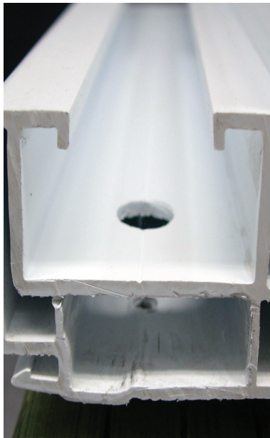
1. Pre-drill window frame.
