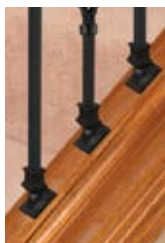
Kneewall Stair Bottom Connection
