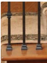
Open Tread Bottom Connection
