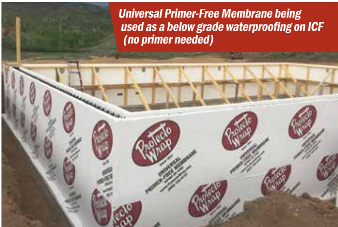
Universal Primer-Free Membrane is being used as Air & Vapor Barrier where the dew point has been engineered to the exterior of the building envelope
