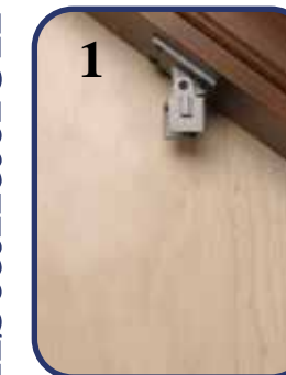
Install Clip To Handrail and Tread
