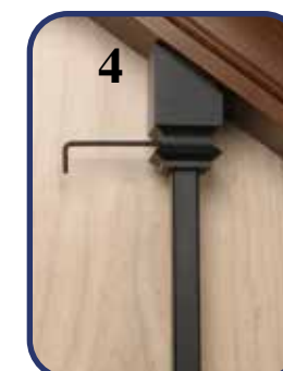
Slide Shoe In Place And Tighten
