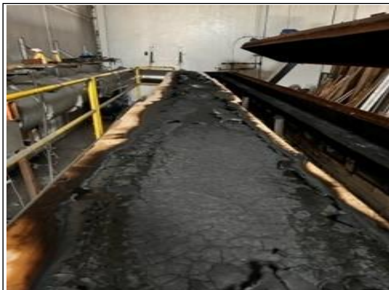
Photo No. 2 Post Test
