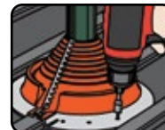
5. Fasten Retrofit to roof
