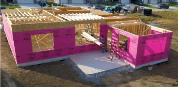
The PINKWRAP® weather barriers are engineered for efficient installation thanks to its semi-transparency, strong tear resistance, wide size, and light weight. Its woven structure offers water resistance with breathability.
