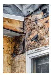
STONEfaçade is the only product on the market that has a true integrated rainscreen. That's essential because moisture intrusion on the exterior wall is one of the leading reasons for wall assembly failure – and costly call backs. Our integrated rainscreen is designed to allow adequate airflow behind the panel. This promotes drying and helps eliminate potential moisture issues like mold and mildew within the wall cavity.
