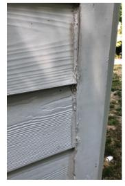
Traditional corners require caulk, which over time can shrink and gather dirt, leaving the substrate prone to water damage.
