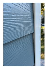
AZEK J-Quick Corner encases the siding to ensure ends are covered with no additional caulk needed.
