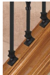
Kneewall Stair Bottom Connection
