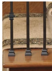
Open Tread Bottom Connection
