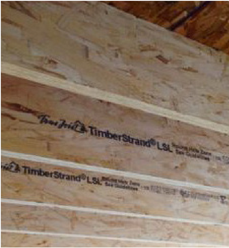
TimberStrand® LSL Floor Joists
