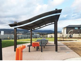
As part of a \$440k upgrade of the Oakbank Boulevard park and playspace, designed by CDA design group for the City of Whittlesea, Stoddart were engaged to supply a centrally located picnic shelter and picnic settings to the project. Stoddart designed, engineered, and fabricated the custom timber wave shelter to suit a 6x6m covered area, as well as providing two Town & Park Metro table settings.
