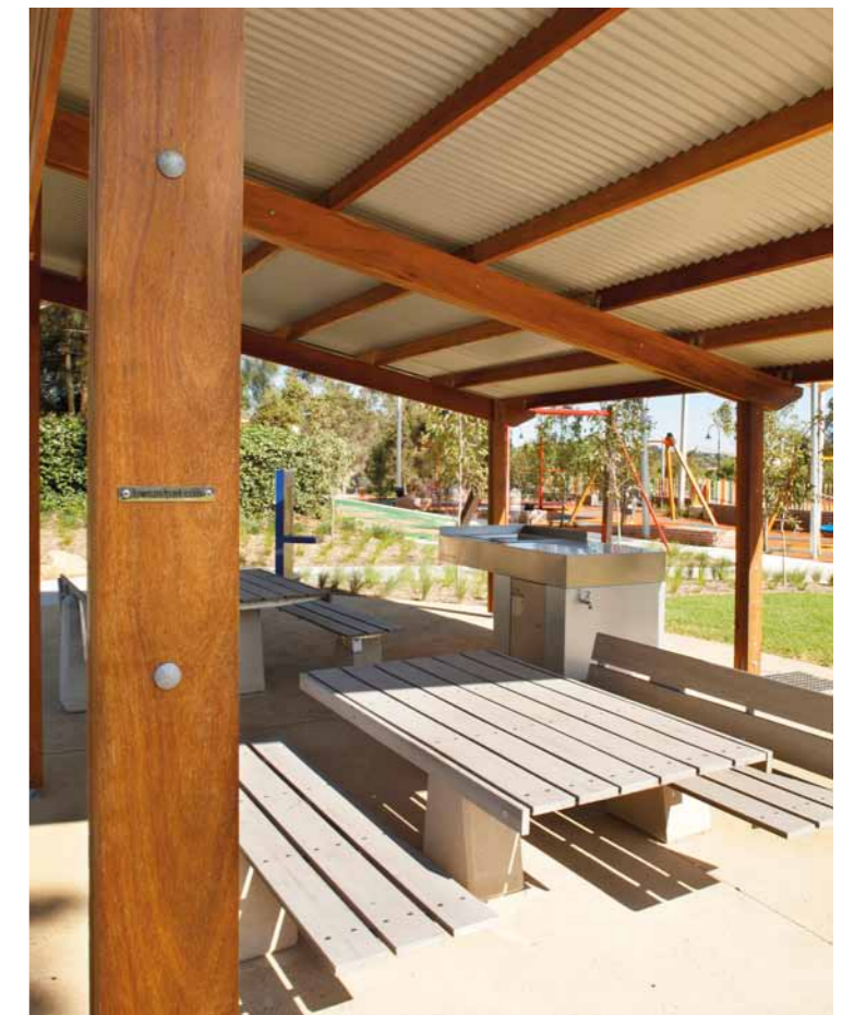
PARKSHELTER The shelter originally specified didn't allow space around the furniture and barbeque for wheelchair users. We designed a new shelter, removing the three centre posts to create circulation space and chose a stronger species of timber to accommodate the increased spans of the new design. Problem solved!
