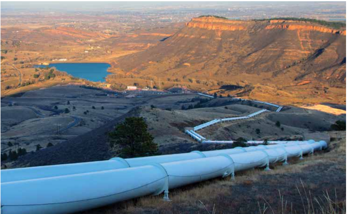
The Flatiron Penstocks above Flatiron Reservoir in Larimer County bring water to Carter Lake and Horsetooth Reservoir via the Colorado-Big Thompson Project.
