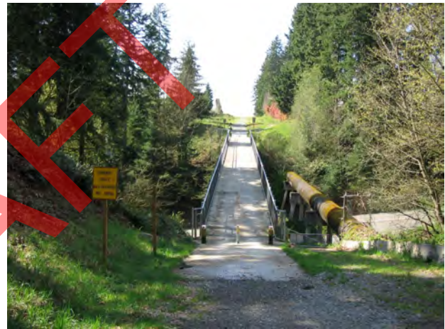
Trail bridge on pipeline greenway in King County, WA.
