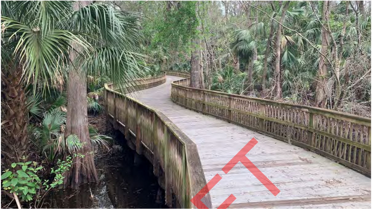
Figure 30. Greenway boardwalk providing access through low-lying natural area
