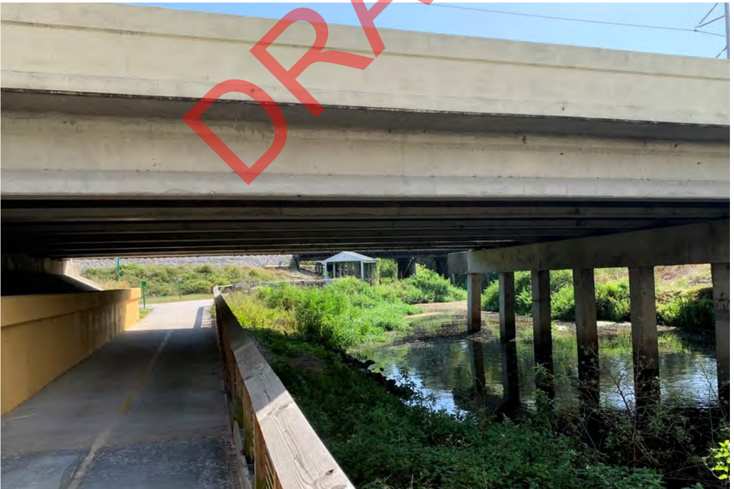
Figure 24. Roadway bridge span accommodating both the greenway and natural stream corridor
