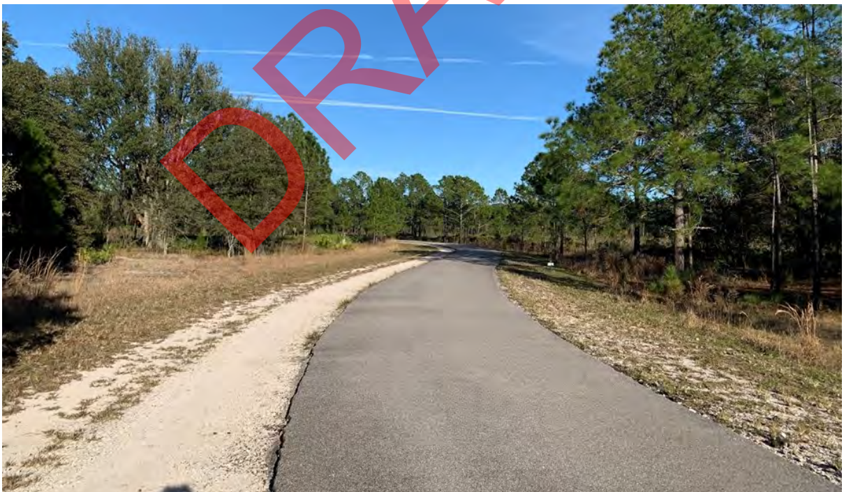
Figure 31. Parallel paved and un-paved greenway surfaces for different user groups
