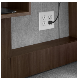
Wall access panel
