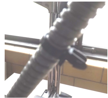
WRAP THE WIRE CLIP AROUND THE CONDUIT BEFORE INSERTING INTO THE POST
