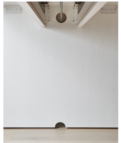
Discreet Wire Cutout on Outside Base Panel
