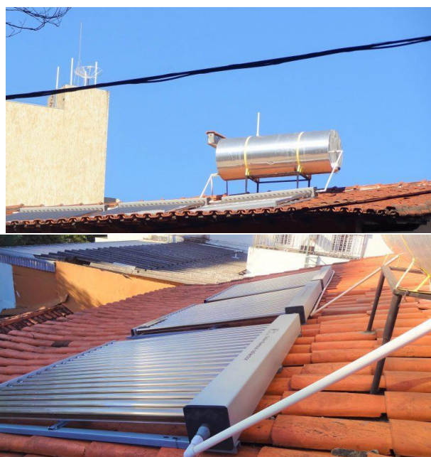
Photos from the already implemented system in the HI Brazil hostel Adrena Sport Hostel, Belo Horizonte.
