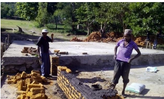
Locals working on the walls of 1 st set of classrooms
