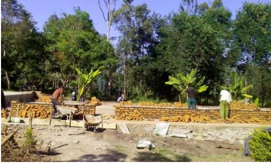
Work on the walls of 1 st set of classrooms
