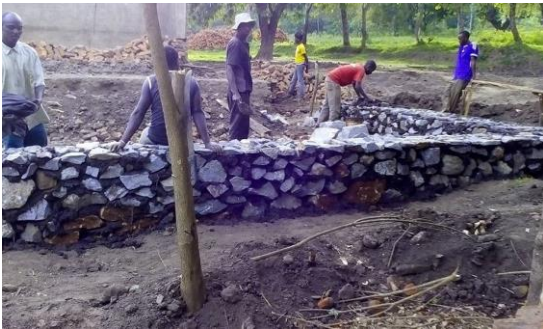
Work on the foundation of next set of classrooms
