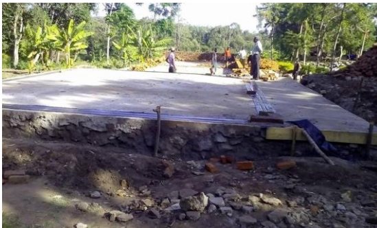
Foundation 1 st set of classrooms completed
