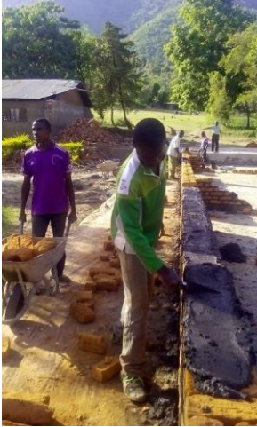
Locals working on the walls of 1 st set of classrooms
