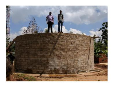
Here you can see that the foundation for the 135,000-liter tank in Gajal is done and walls are already being raised:
