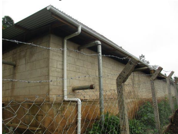
Gutter of the tank in the hills
