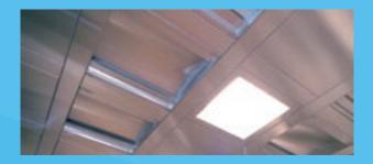
Modifications and options of the Cyclocell cassette ceiling include vertical service columns, fire suppression, and trim around the elements. The system can also incorporate emergency lighting and fire-rated enclosure.
