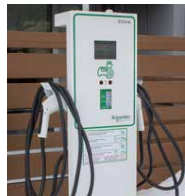
Electric Car Charging Station
