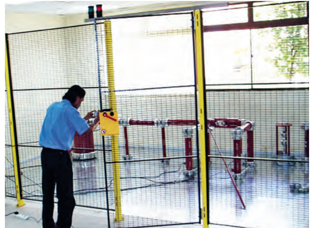
Installation of Safety Fence
