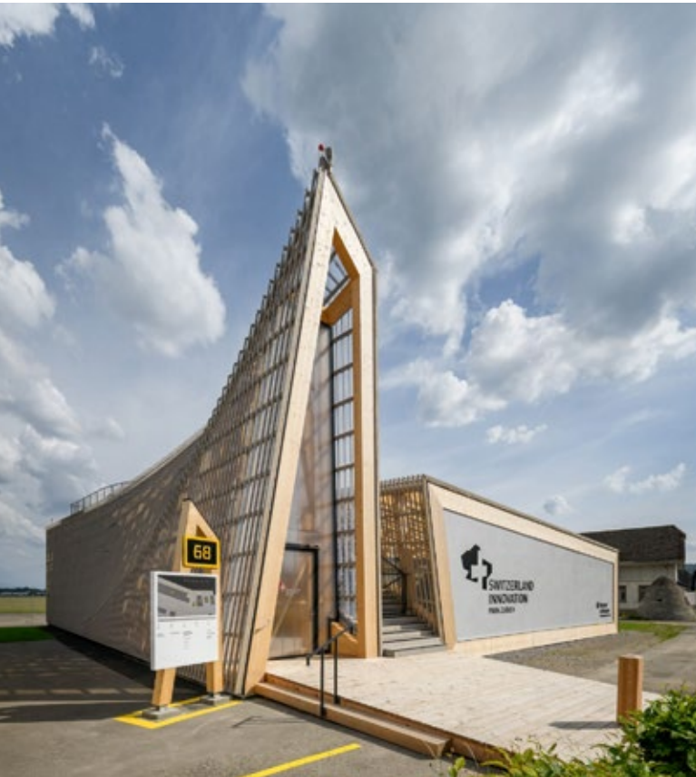
Corporate office of the Innovation Park Zurich Foundation
