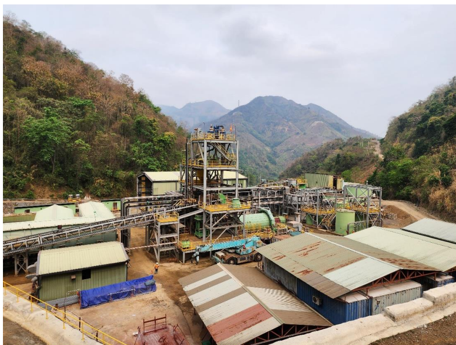
Figure 41: Historical Ban Phuc processing plant.
