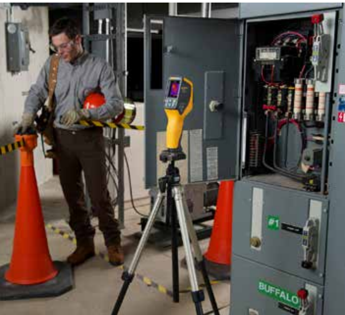
Automated monitoring alarms available on the VT04.
