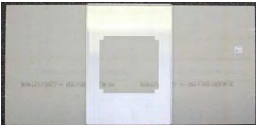
Figure 4: Ceiling Tile Brace on ceiling tile
