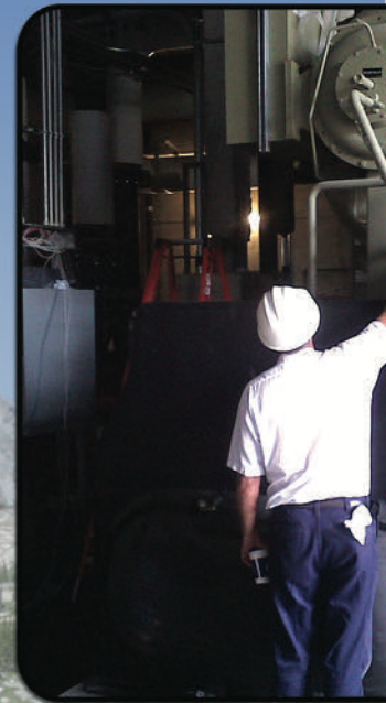
Above: This 2,000 ton system was evacuated from 2,000 microns atmosphere to 1,000 microns in 1 day instead of days with a belt driven pump.
