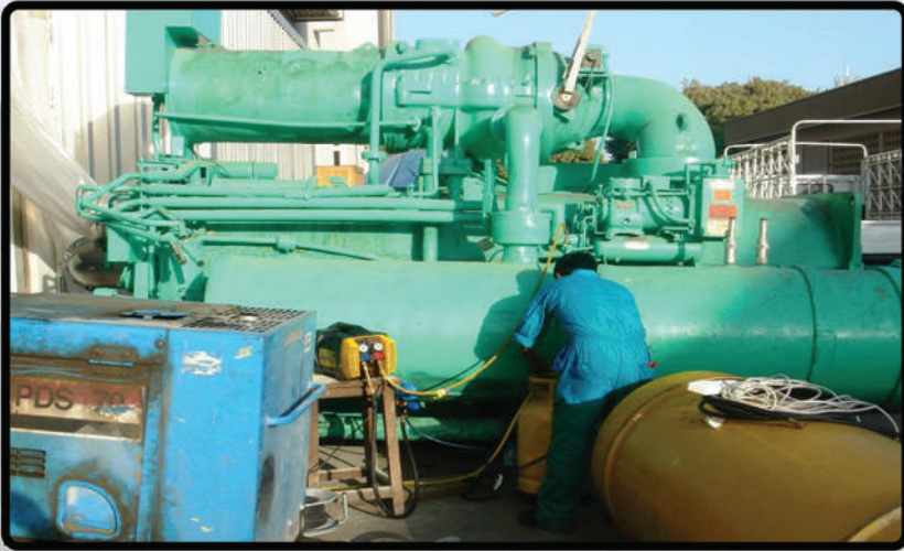
Above: Chillers containing 4000 lbs. of R134a being recovered with a G5Twin in the sweltering heat of Saudi Arabia. What once took a week now takes only 18 hours with the speed and reliability of the G5Twin.
