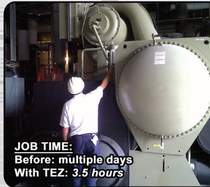
Above: This 2,000 ton chiller was pulled from atmospheric to 1,000 microns in only 3.5 hours, instead of days with a belt-driven pump.
