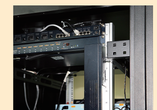
5. Z bracket, mounting style 2
