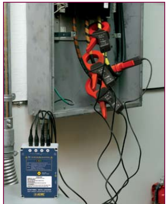
Model SDL A402 recording phase and neutral currents on a feeder.
