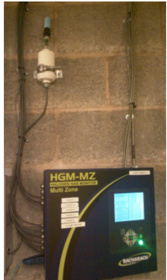
Figure 7. Indoor Filter Mounting Example
