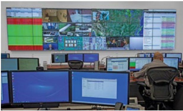
▲ American Water's control room display wall comprises 21 ultra-narrow bezel LCD flat panels from Christie.
