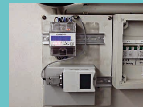
Datalogger S7021 reads and records data from electrometer.
