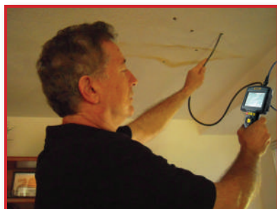
Inspecting a crawl space the quick and easy way
