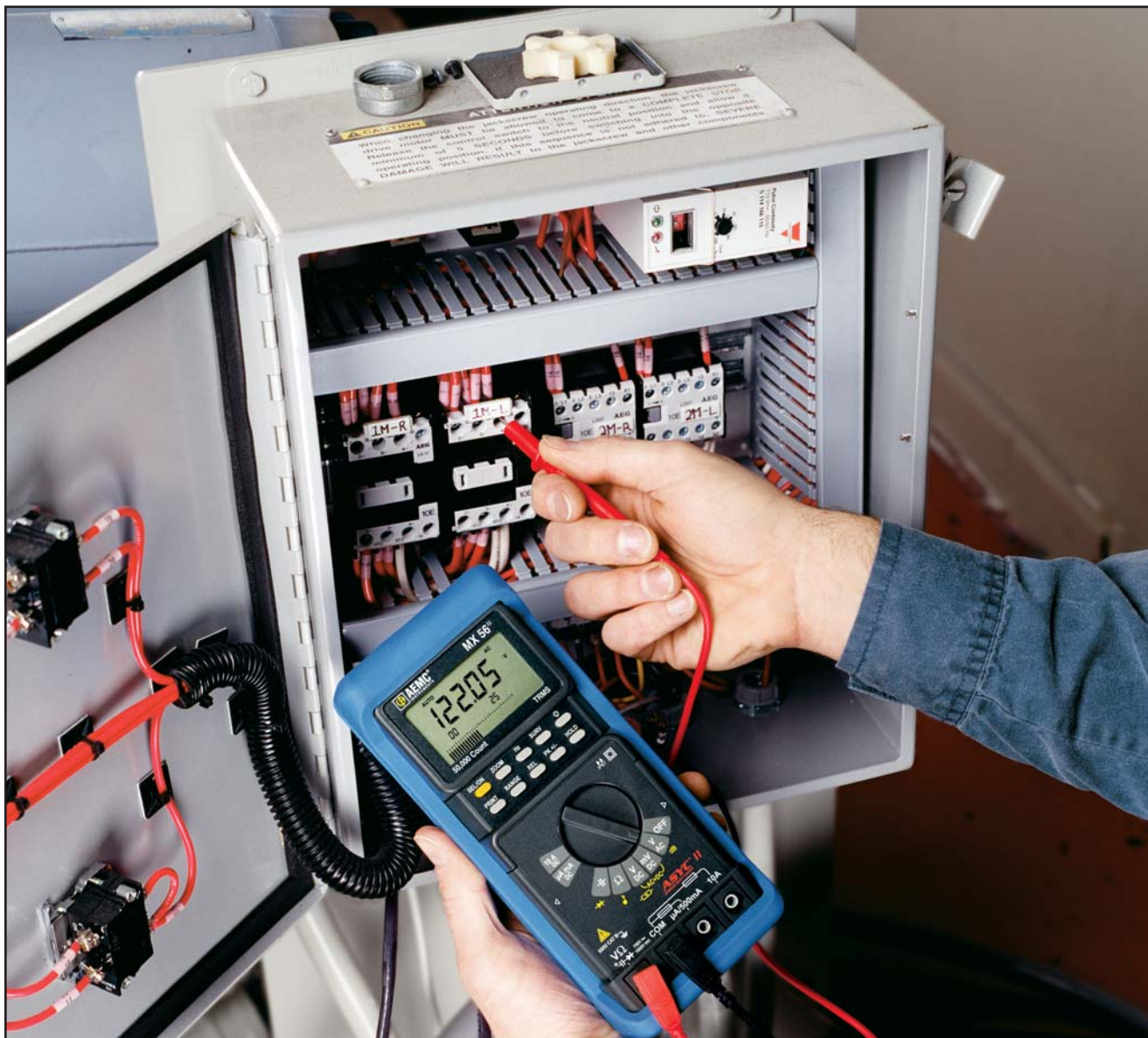
Model MX56™ measuring DC voltages in a signal control panel.
