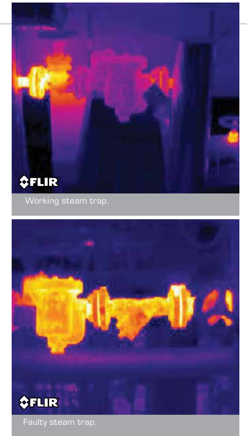
Energy Loss Discover missing insulation, faulty HVAC systems, and other issues that waste energy and lots of money.
