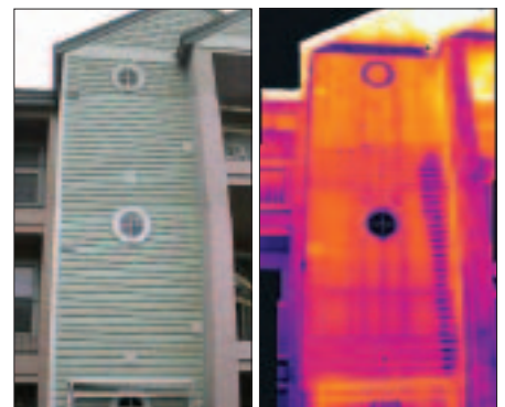
The thermogram of this vinyl-sided 3-floor apartment house clearly shows the path of a serious leak from a washing machine on the third floor, which is completely hidden within the wall.
