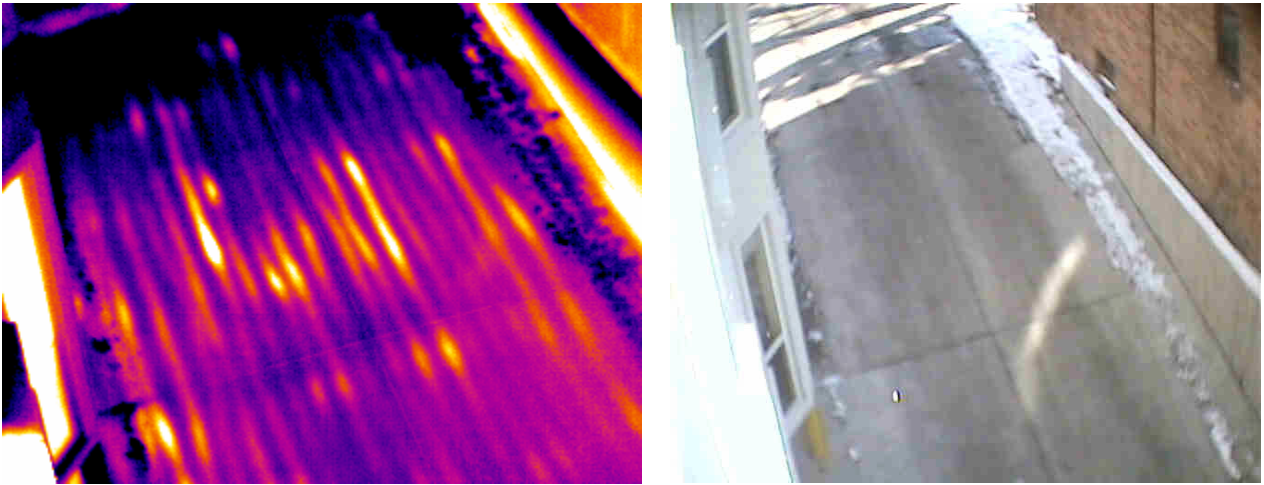
Figure 6. Note differential heating of lines indicating multiple variances in radiant heat line depth below the surface of the concrete.
