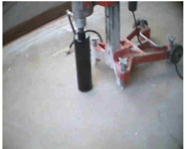
Figure 8. Concrete coring saw positioned between radiant heat lines to prevent damage to the system and subsequent leakage.
