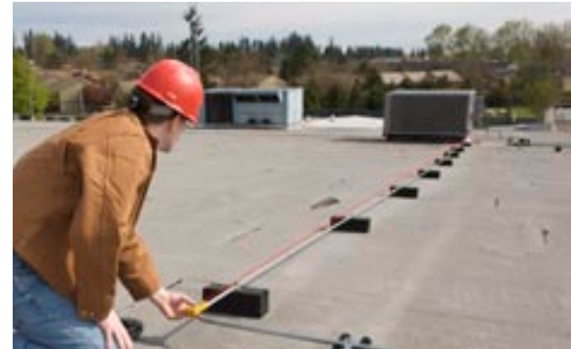
Measuring long conduit runs.
